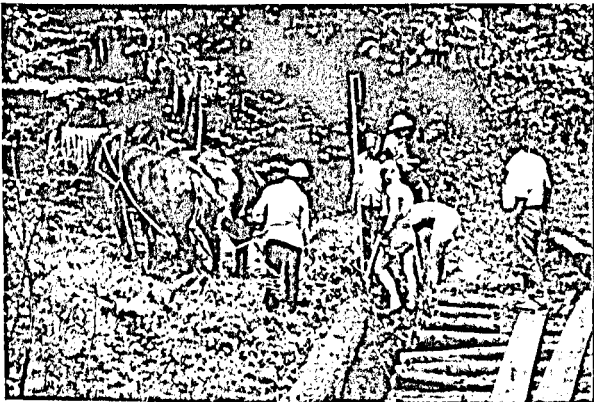
Supervising the work
